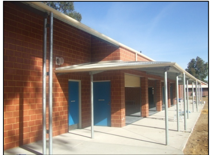
New Covered Assembly Building
